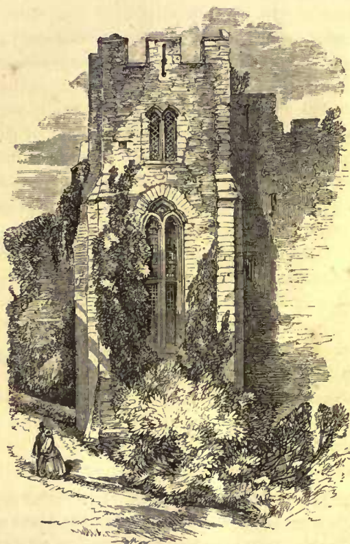
A TOWER IN CHEPSTOW CASTLE.
